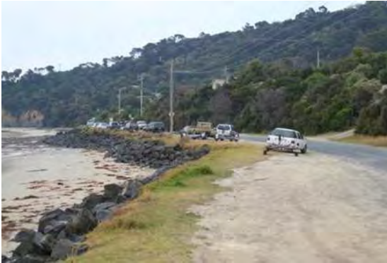
Figure 4: Existing erosion control works and parking near Hall
